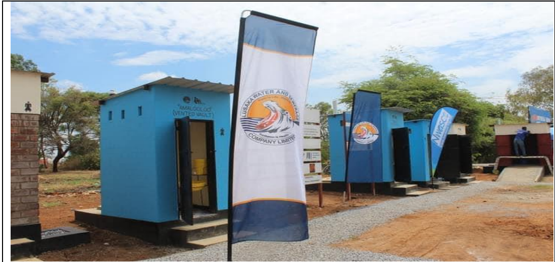
Figure H: Newly Constructed Toilets
