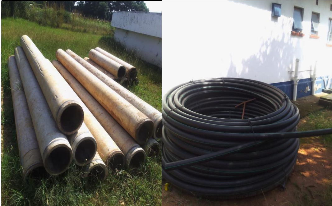
Figure 4.9: Types of pipes in the study area (LHS: Asbestos pipes; RHS: Poly pipes). (Source: Field data, 2022).
