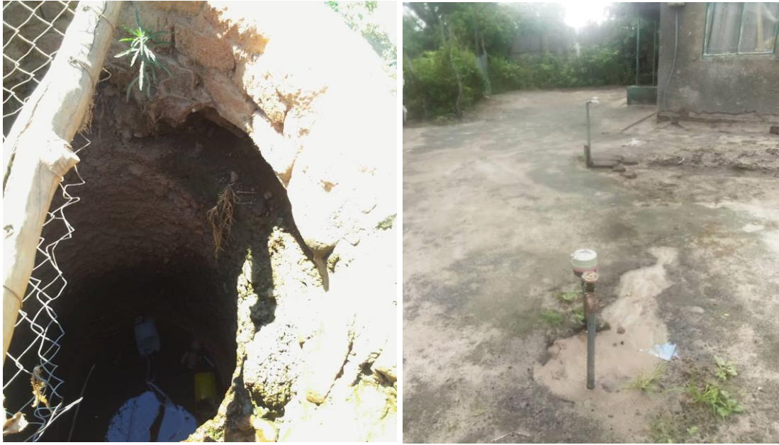
Figure 4.5: Condition of water points from the study area (LHS: A dug well; RHS: A tap). (Source: Field data, 2022)
