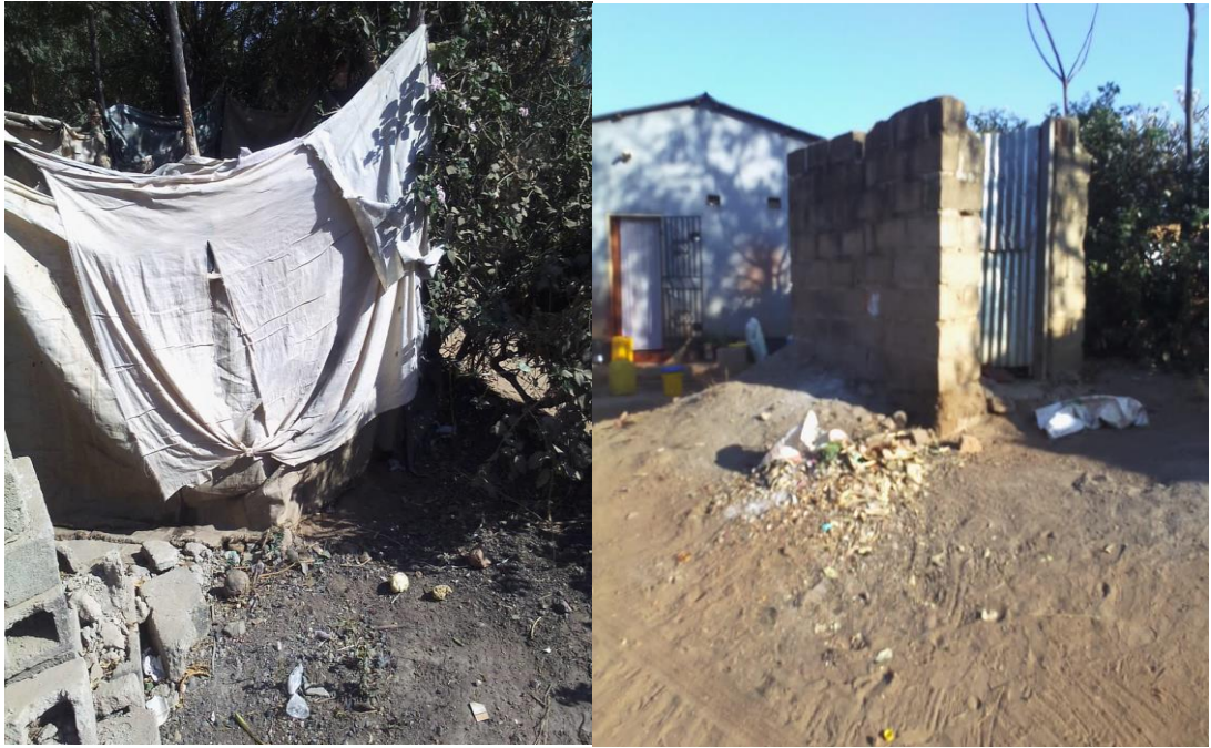
Figure 2 Types of toilets in the study area (LHS: Temporal pit latrine without concrete slab; RHS: Semi-permanent pit latrine with concrete slab). (Source: Field data, 2022).
