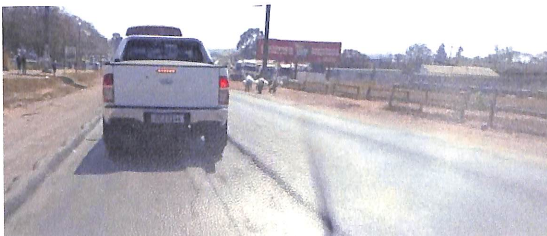
Fig. 38. An example of the ridges in the tarmac created by heavy trucks. 2019.
