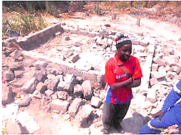
Fig.120: Mr Kampelembe's house demolished to make way for the mine but with a modern replacement to move into. Credit: Jack Zimba's blog spot, 2014.
