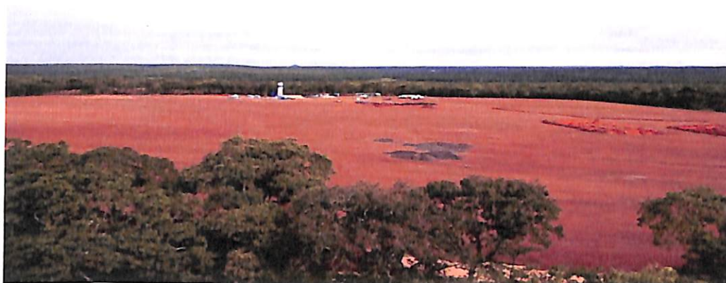
Fig. 69: Clearing of the site, early 2006. Source: Craig Williams' power point, 'The Story of Lumwana', 2012.
