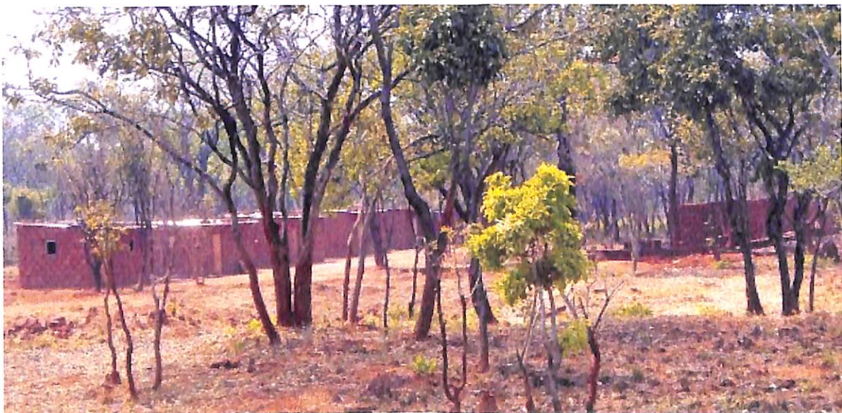
Fig. 135: On the edge of the T5, before Kalumbila turn-off, another entrepreneurial project- the building of rooms to rent in anticipation of the influx, 2014.
