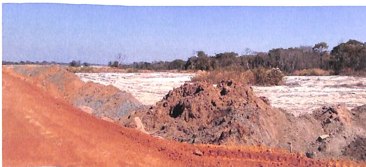
Fig. 65b: New Kalumbila tailings spreading out with bulldozing to build containment walls, 2019.
