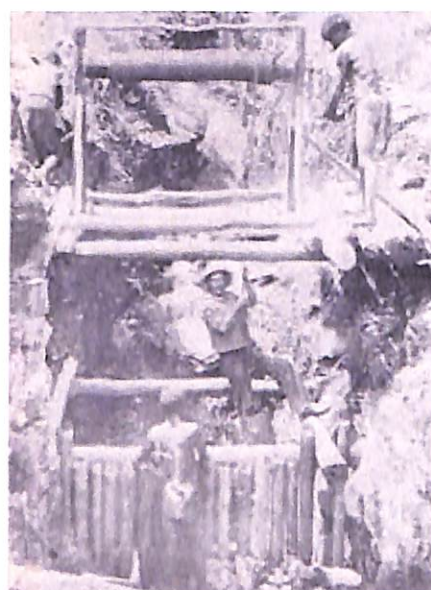
Fig. 6: Early colonial workings, Kansanshi mine, 1901. Credit: National Archives of Zambia Zambia (NAZ).
