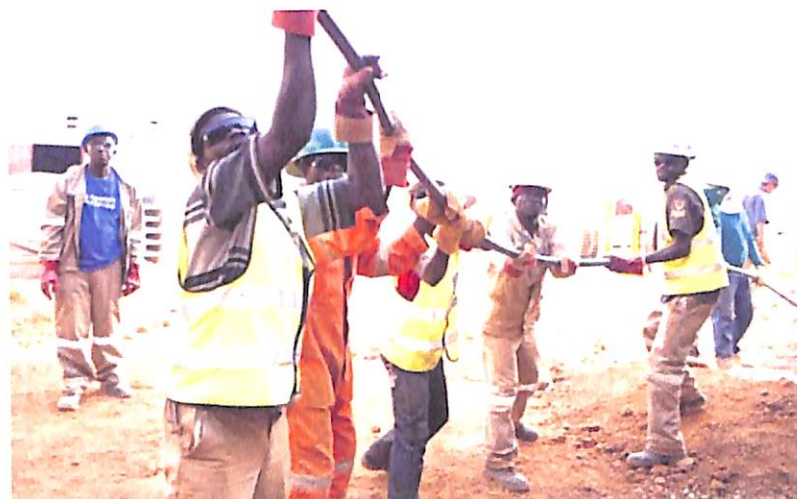
Fig. 145: Cable pulling by locals, during the construction phase. Credit: Trident power point, Jan. 2014.
