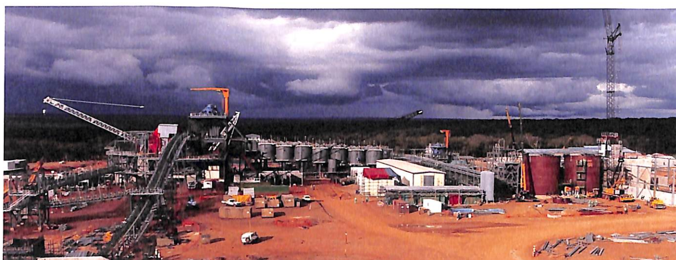
Fig. 70: Lumwana mine, on track for completion mid-2008. Source: Craig Williams' power point, 'The Story of Lumwana', 2012.
