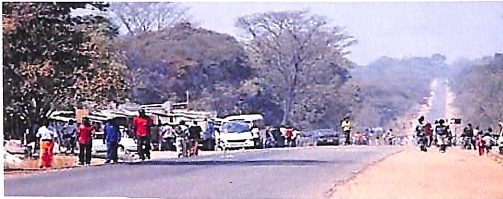
Fig.105: The T5 in the Manyama area, by then a very busy area. Credit: Barrick Beyond Borders, Managing In-Migration at Lumwana, December 2012. (Note the un-supported edges of the tarmac which will deteriorate quickly)
