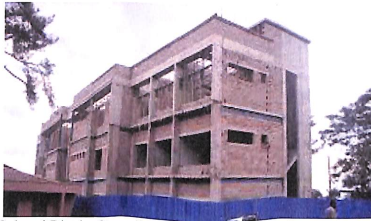
Fig. 53. The new Solwezi District Council building under construction, 2016. Credit: Lusaka Times.
