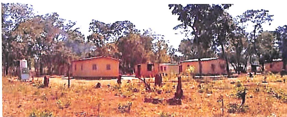
Fig. 129: Southern Resettlement housing.
