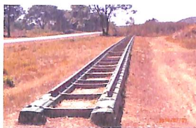
Fig. 30: The demonstration length of rail, besides the T5 near the Chingola turn-off, the only physical sign of the proposed railway, laid for the opening in 2005, pictured in 2012.
