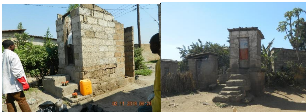
Figure 4-3: Examples of pit latrines with elevated latrine vaults (Source: This study)
