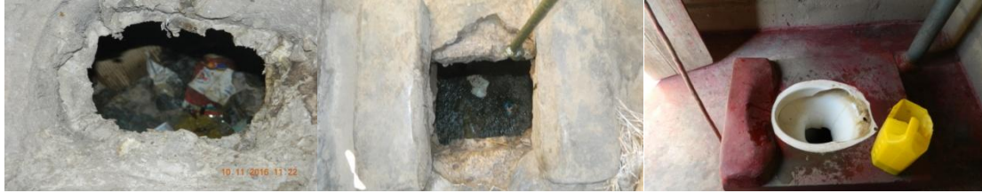
Figure 5-1: Example of interfaces that discourage direct latrine usage by children (Source: This study)
