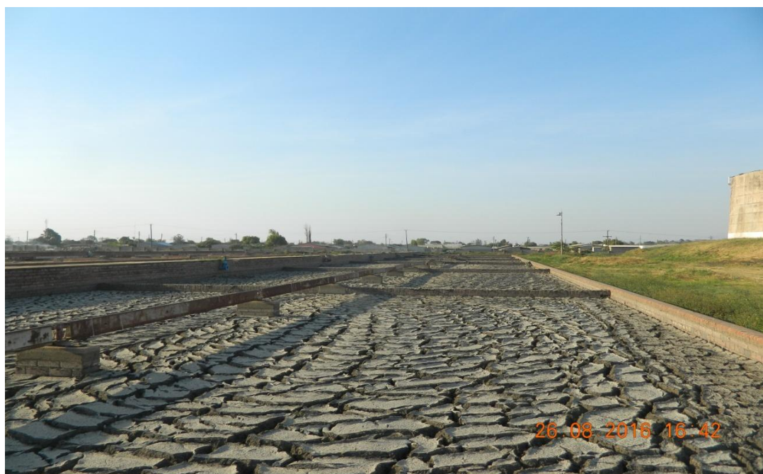
Figure 2-7: Sludge on drying beds at Manchinchhi Wastewater Treatment Plant (Source: This study)
