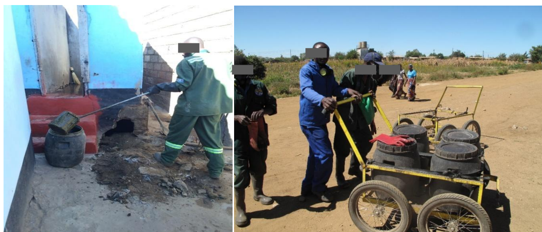
Figure 2-5: Faecal sludge emptying and transportation (LHS: Scooping of sludge from a pit latrine through a hole on the side; RHS: Transportation of sludge using a hand cart)(Source: This study).
