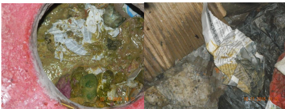
Figure 4-7: Pit latrine contents showing presence of solid waste (Source: This study)
