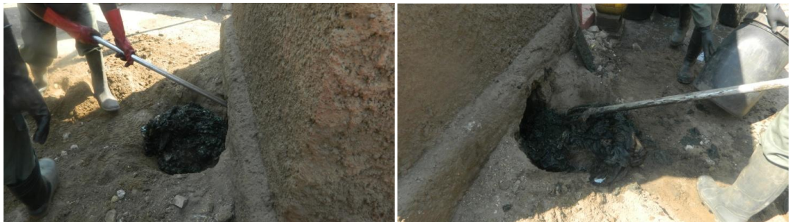
Figure 5-2: The pit latrine desludging process (Note the possible mixing of the sludge with the loose sand from the newly dug pit) (Source: This study).
